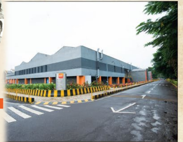
▲ GSK India's present-day manufacturing factory located in Nashik, Maharashtra
